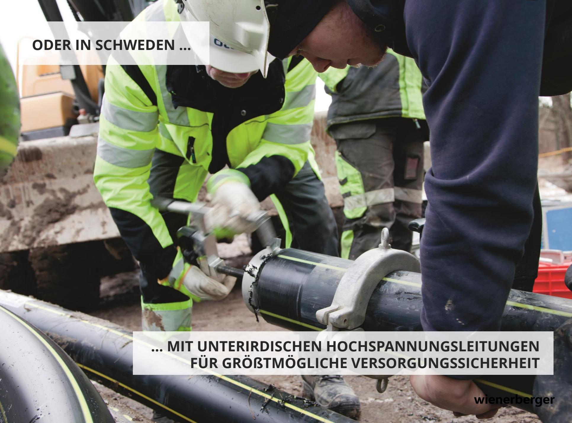
A photograph showing construction workers in high-visibility yellow and black safety gear working on large black underground cables. One worker in the foreground is using a tool to strip the outer layer of a cable. Another worker in the background is also visible. The scene is outdoors, likely at a construction site for underground power lines.
